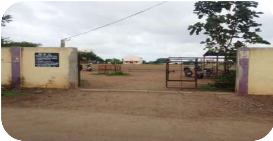
Second Entrance Gate
