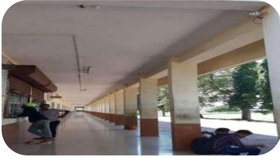
Front Side CCTV
